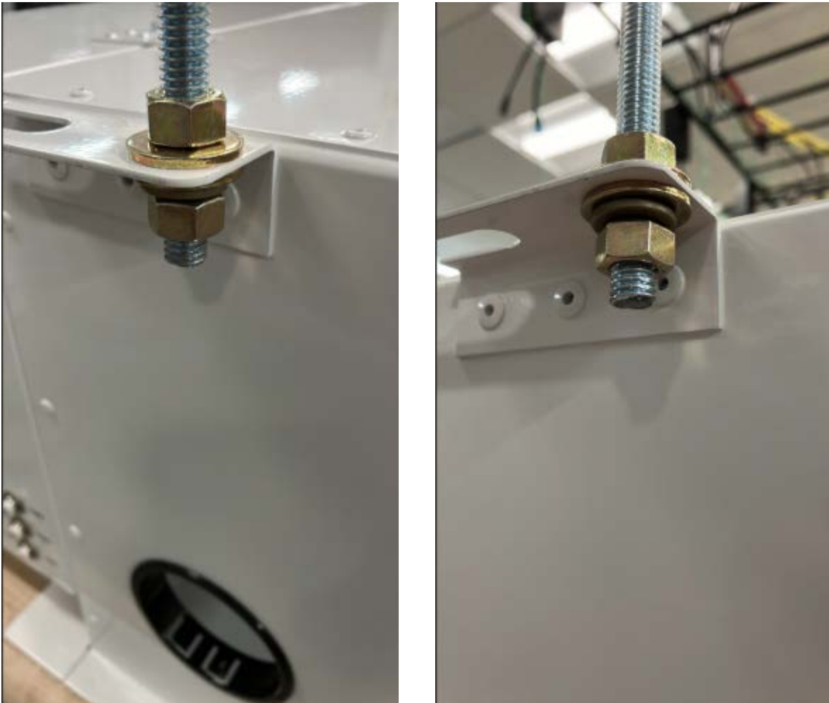
Figure 7. Down Rod Assembly Supporting Edge Enclosure
