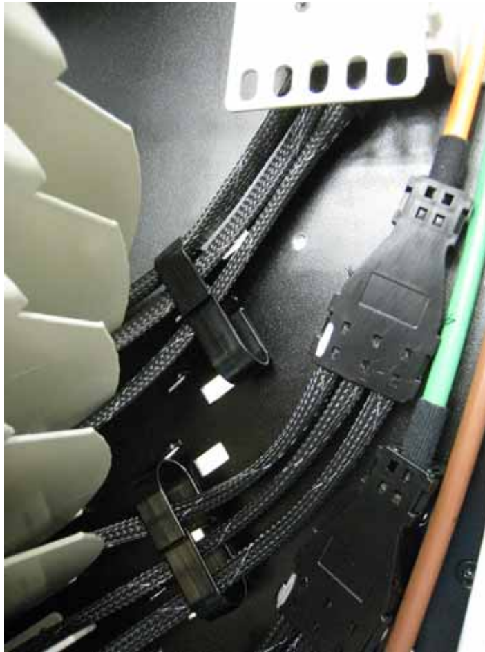
Figure 11. OSP Mesh Sleeves Within Clips and Routed to Shelves
