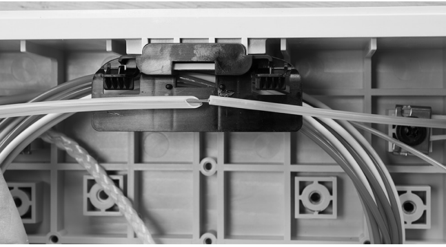
4.3.7 Insert the fibers into the transportation tube.
