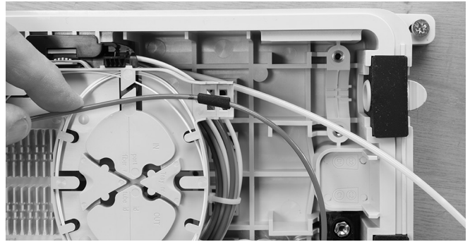
3.3.17 Wrap a piece of foam around the tube as shown.
