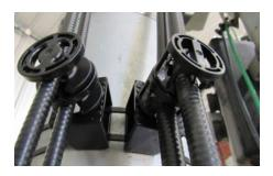
Stack SnapTak hangers into composite adapters such as the SA-1C for PIM-free routing of coaxial, fiber, and power jumpers in seconds
